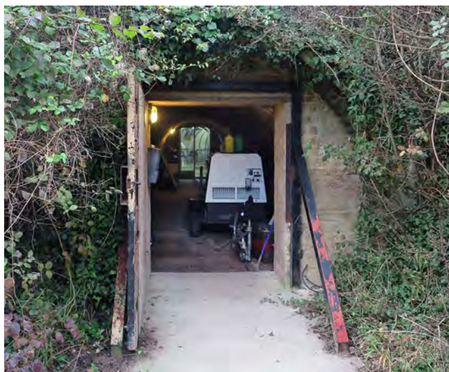
The emergency exit to the WWII tunnels beneath Fort Southwick, where we made our entrance.
